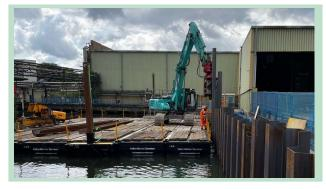
The new fish pass will be built in much the same way as the weir rebuild, within a sheet piled cofferdam, but will require deep excavations within the footprint of the existing weir to create the resting pool, and the construction of new reinforced concrete walls to support the structure and form the inside surface of the pass. Only when the new fish pass is completed will the existing pass be closed to flow and the new canoe portage steps poured.
